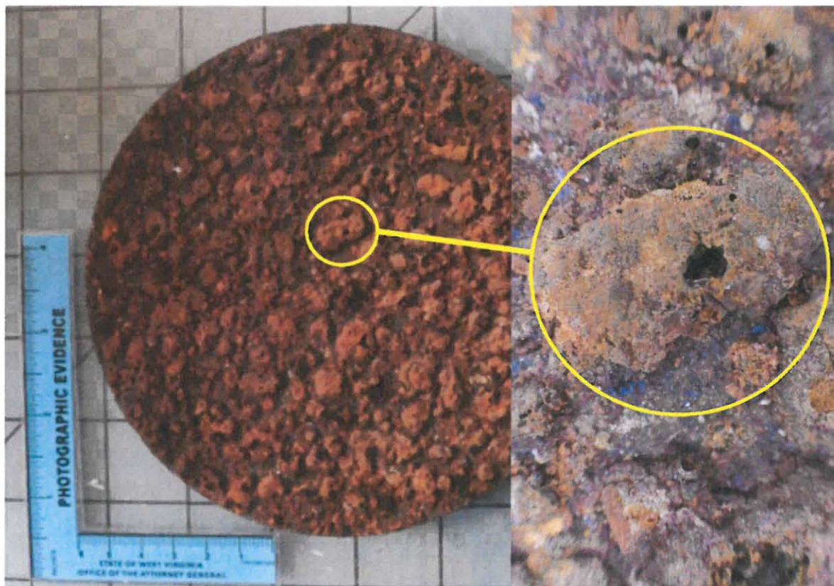
Corrosion on inside of coupon removed from side of tank 396
