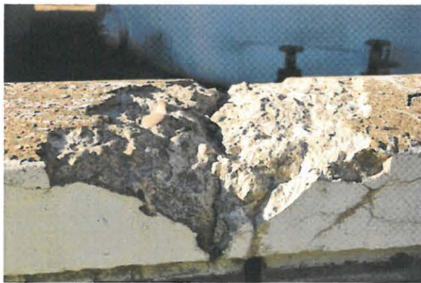
Cap of brick containment wall facing Barlow Drive
